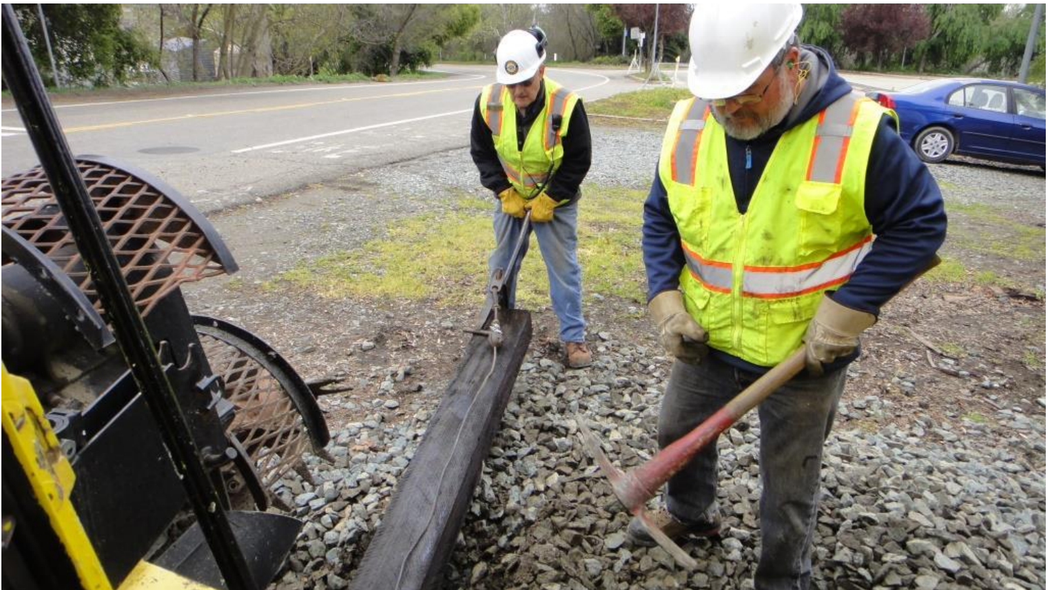
Mike W. connects the inserting cable to the tie as Steve W. digs a bit out from under it
