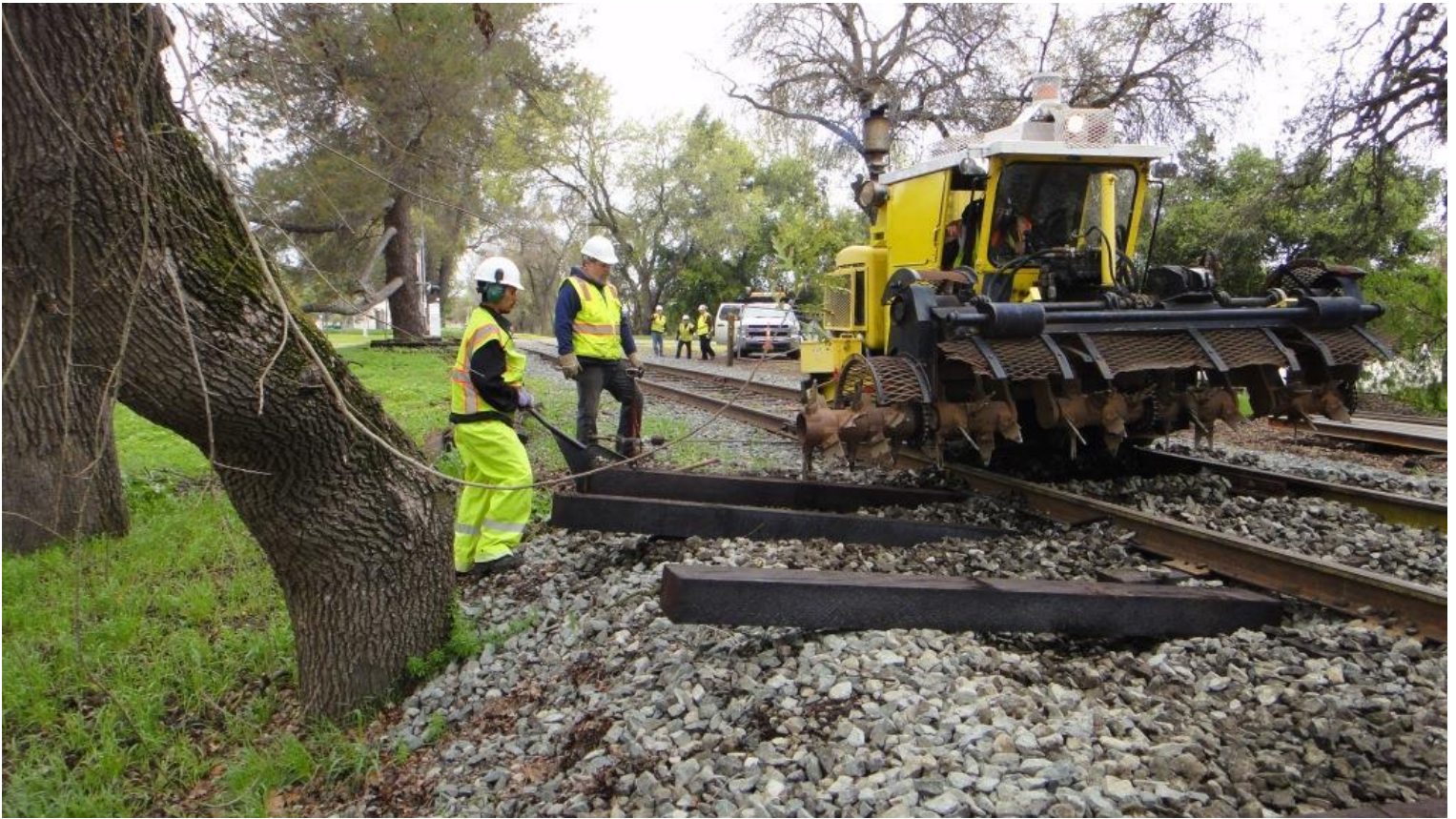
Using the inserter function on the scarifier, Mike F. in the scarifier pulls in a tie guided by Josh
