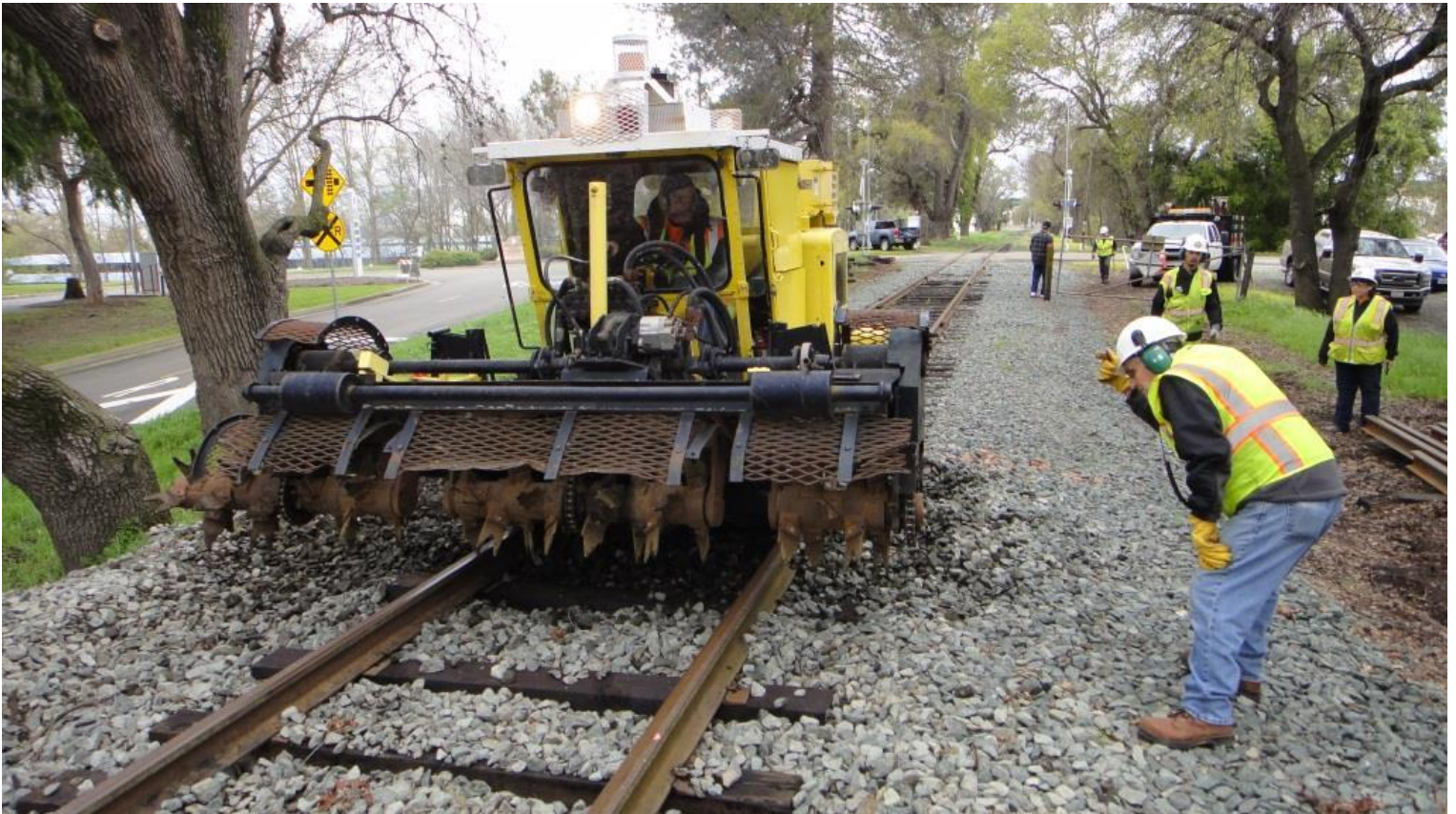
Mike W. provides guidance to Mike F. in the scarifier to line him up
