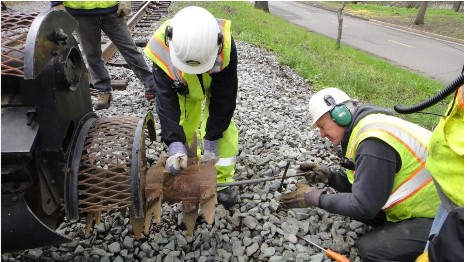
Josh holds the extension-drum in place while Steve N. tightens its bolts
