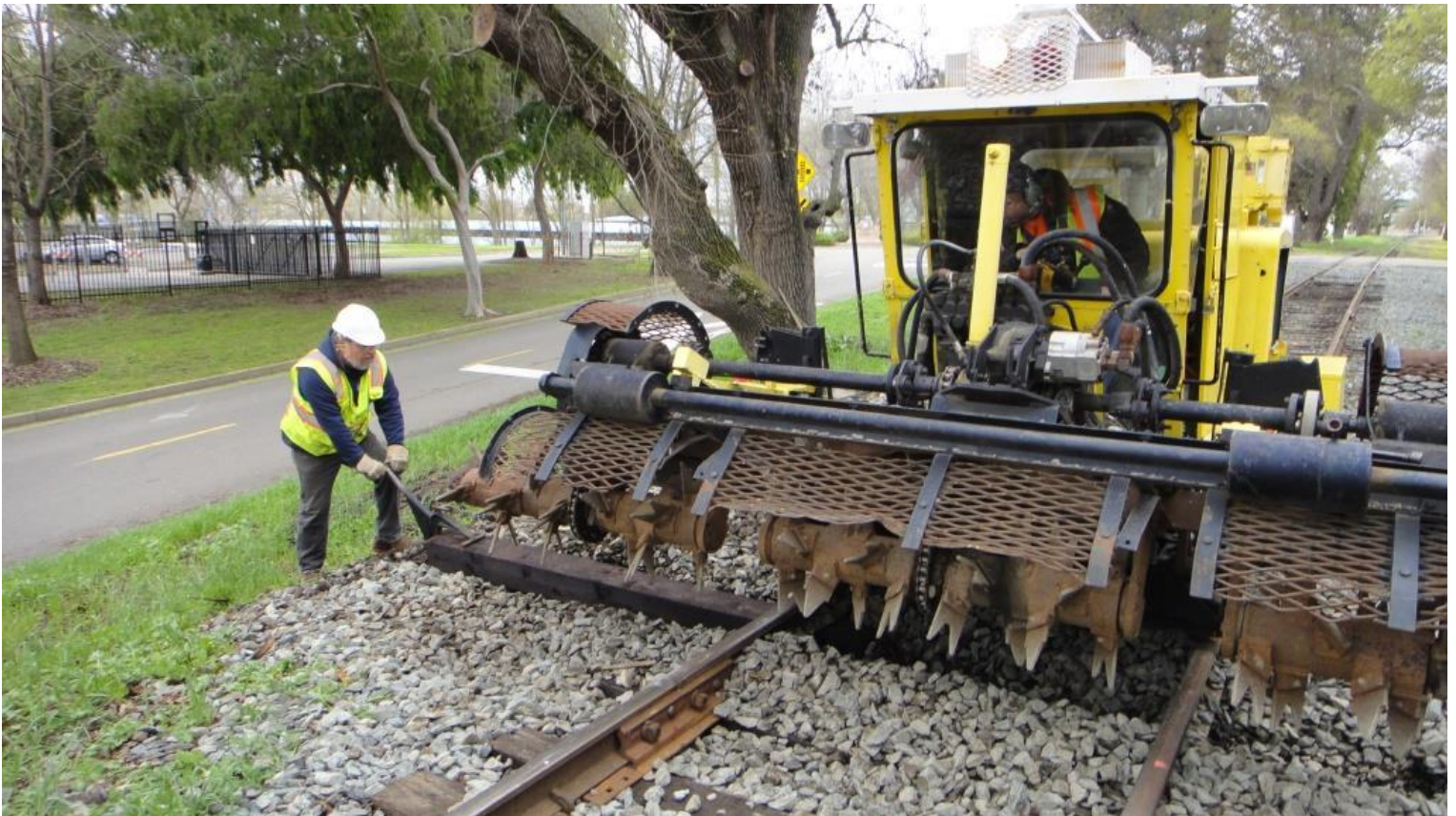
Steve W. guides a tie in place
