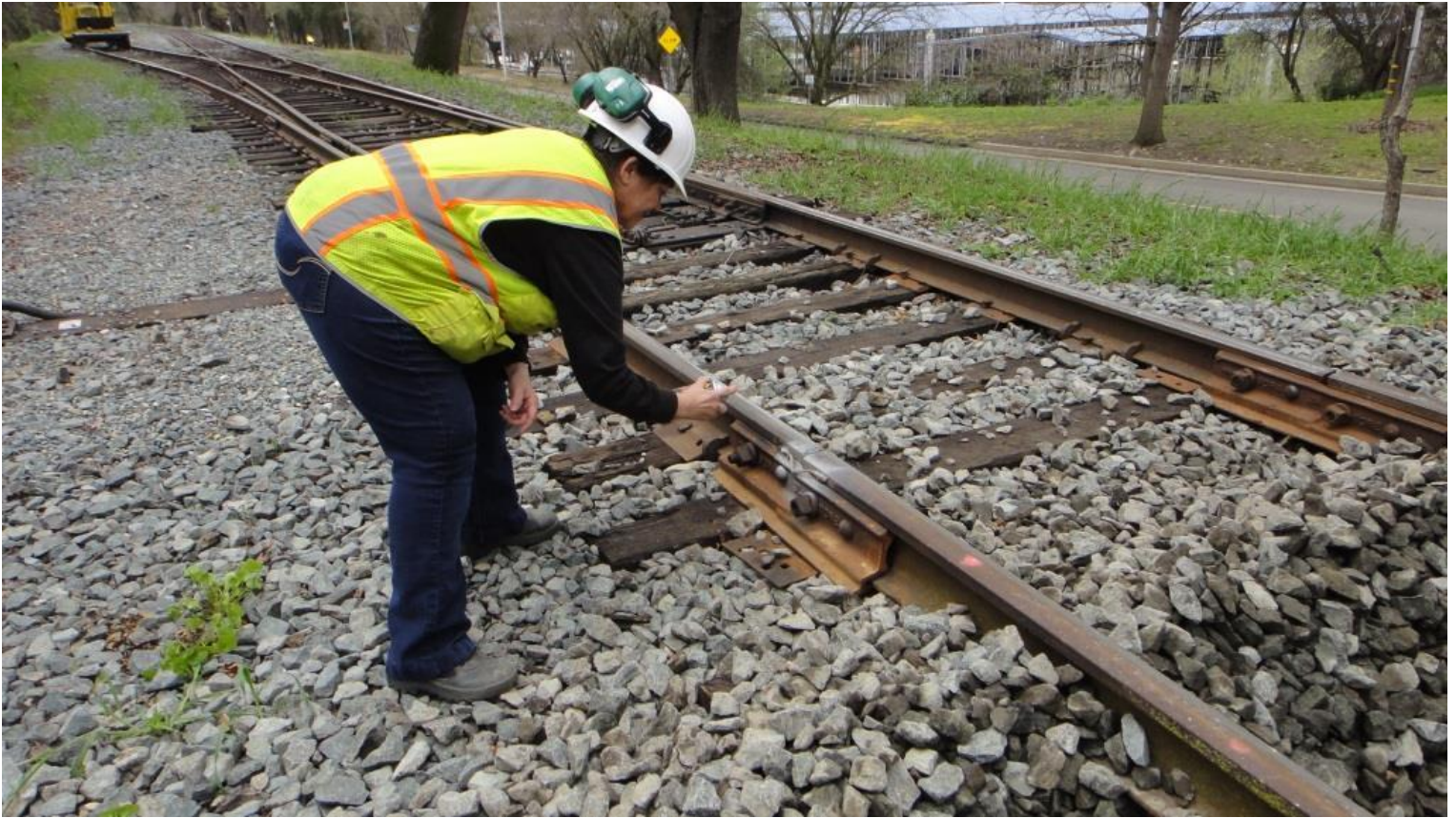
Pam, on shine-removal patrol, paints the bright copper bond-wires a dull shade of gray
