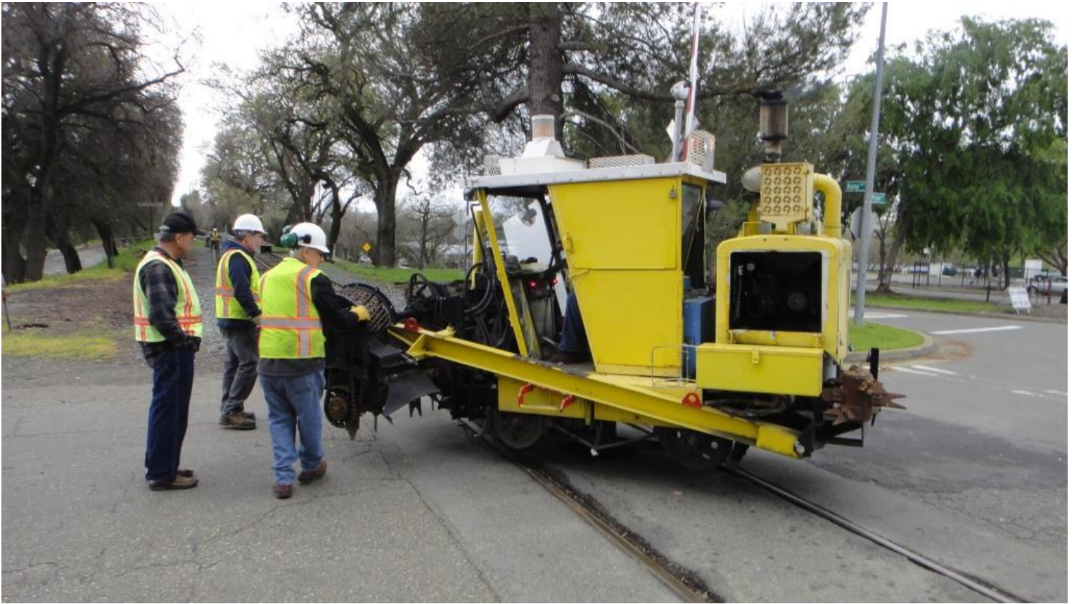
As the scarifier is spun, Mike F. takes an "E-ticket" ride
