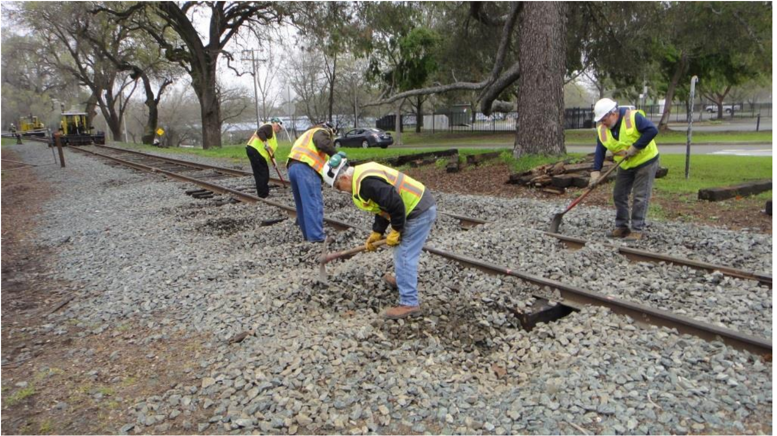
Harry, Mike F., Mike W. and Steve W. fill in holes in the ballast as the rain starts to fall
