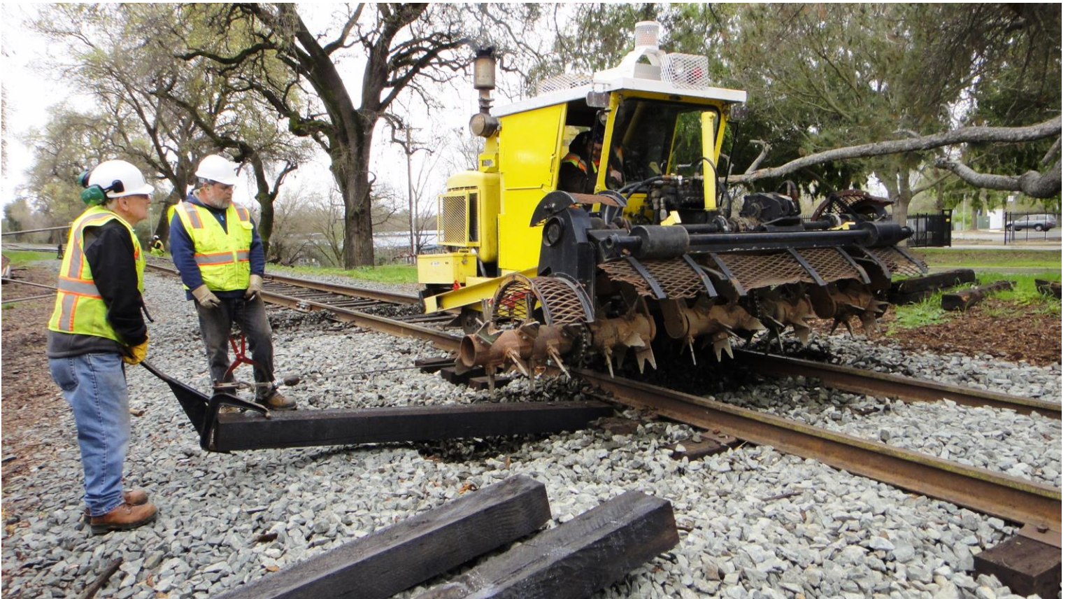
Mike W. guides the next tie into position
