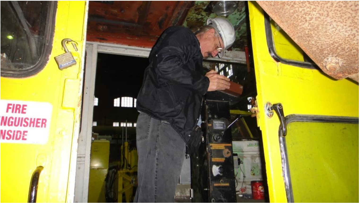
Fred in the cab of the ballast regulator – a.k.a. USS Sea Tiger – making adjustments to the control stand while on the quest for air leaks
