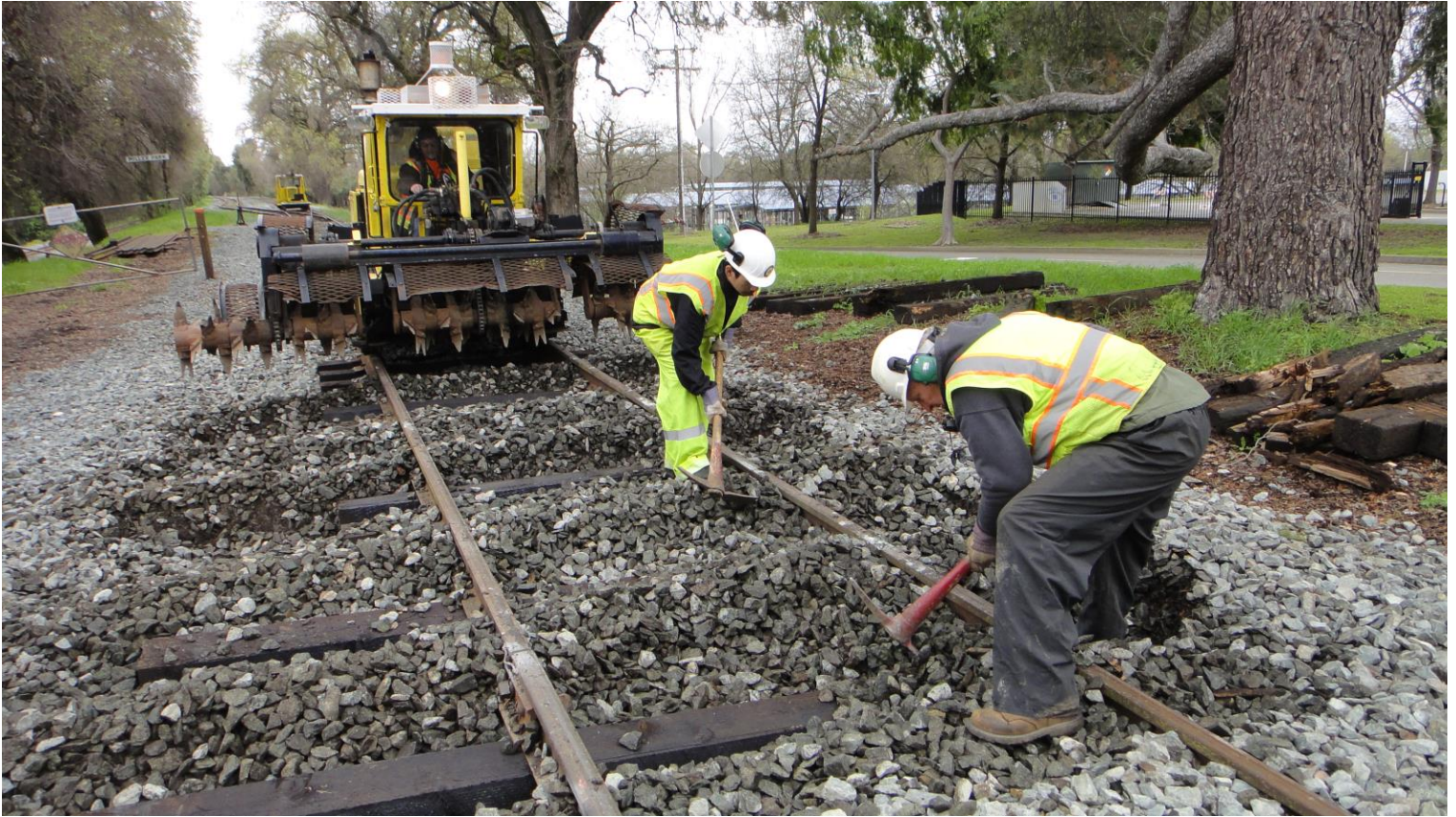
Josh and Steve N. clear a path for the tie by digging out the rock that has bunched-up under the west rail
